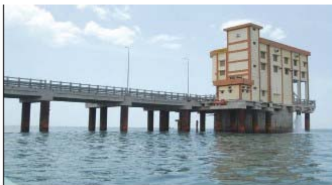
The intake facility of the RO-based desalination plant installed for Chennai Petroleum Corporation Ltd.
